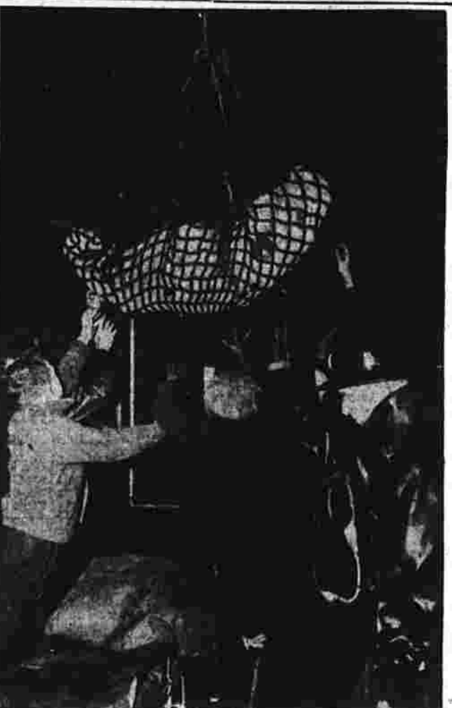
The bodies of some of the 25 known victims of the fire that swept the five-story Terminal Hotel in Atlanta, Ga., being lowered to the ground in a sling after being dug out of the debris in the wrecked building. A stretcher can be seen in the foreground, waiting for the arrival of a stretcher to make various plans.
